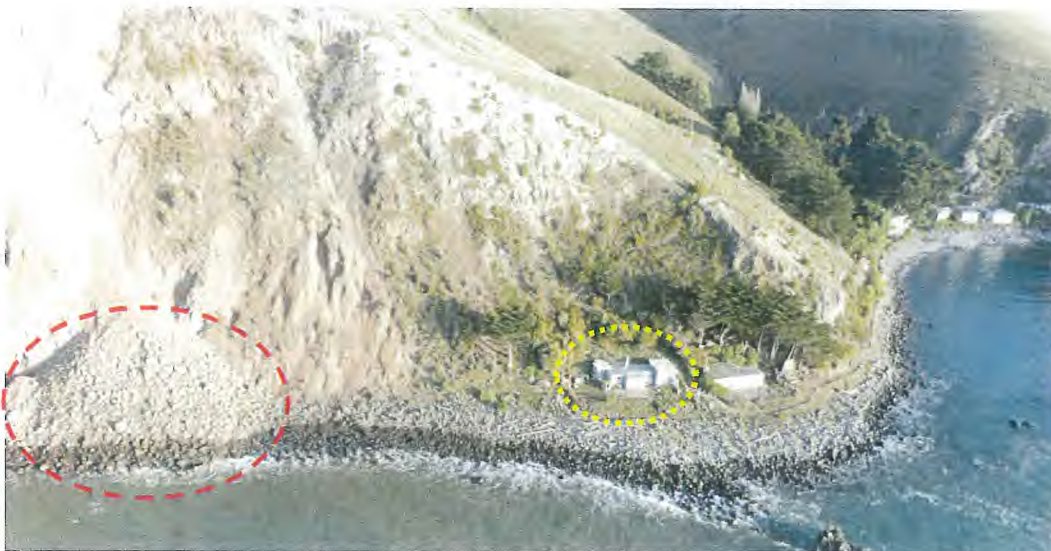
View of 1 Boulder Bay (yellow circle), showing debris from cliff collapse that occurred on 13 June, 2011 (red circle).
