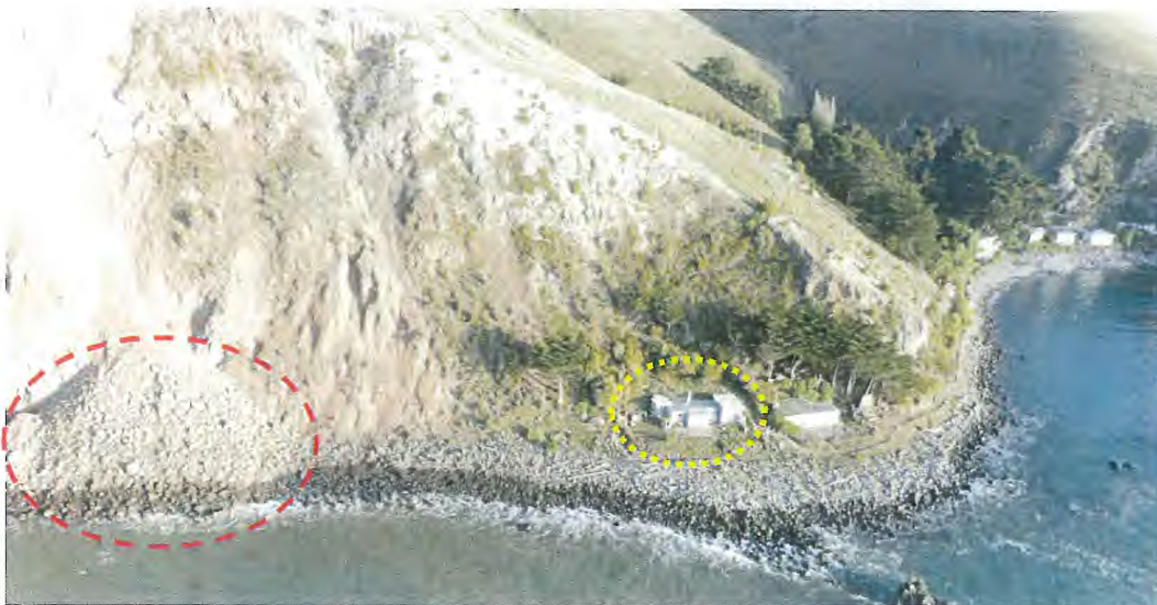
View of 1 Boulder Bay (yellow circle), showing debris from cliff collapse that occurred on 13 June, 2011 (red circle).
