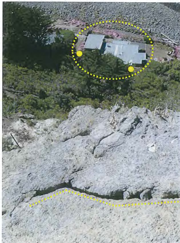
View from cliff top above 1 Boulder Bay (yellow dashed circle). A tension crack (yellow dashed line) is present near the cliff edge. Two boulders (yellow circles) landed near the dwelling following the 22 Feb aftershock.
